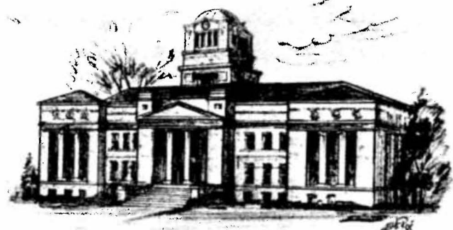
Navarre County Courthouse
