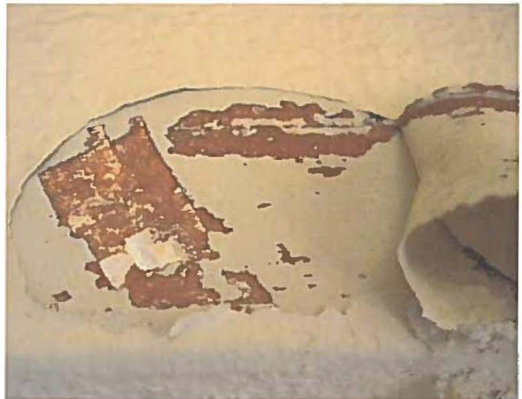
The observation was made that the plaster ceilings of the of the exterior porticos had a first generation of dark red. This was corroborated on the South Elevation where scaffolding allowed access. There also indication that the lower, ground floor porticos were the same red. Though these ceilings are replacements on the ground floors the overpaint is still very obvious.
